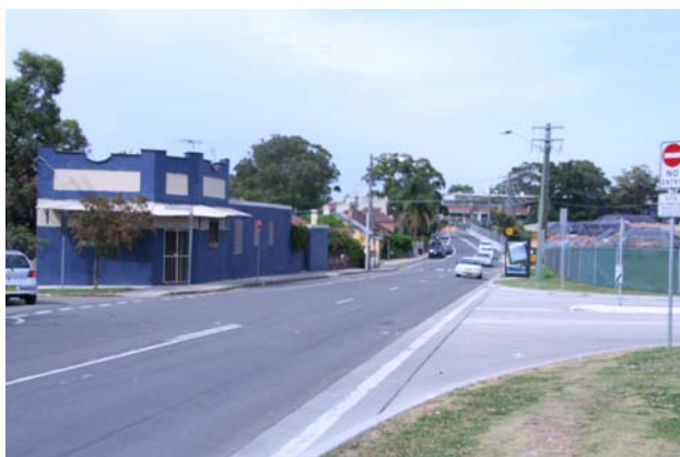
View of Balmain Road, with the existing bus entry driveway on the right.
